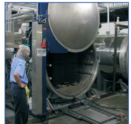
Cage Lift Cage Lift
